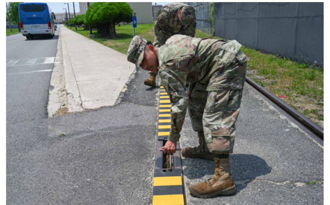
Airman 1st Class Jayden Bolo, 8th Maintenance Squadron aircraft metals technology journeyman, uses a specially fabricated hook to install a custom built railroad track cover they created at Kunsan Air Base, Republic of Korea, June 17, 2025. This enhancement directly contributes to the Wolf Pack's mission readiness by reducing the likelihood of railroad track-related safety incidents that could render personnel non-mission-capable. ▲
